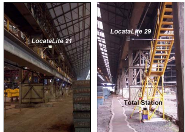
Figure 6. Example installations of LocataLite antennas and total station used for 'truth' positions.
