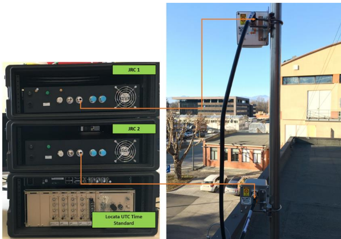
Figure 3-14: Building 72C Installation
