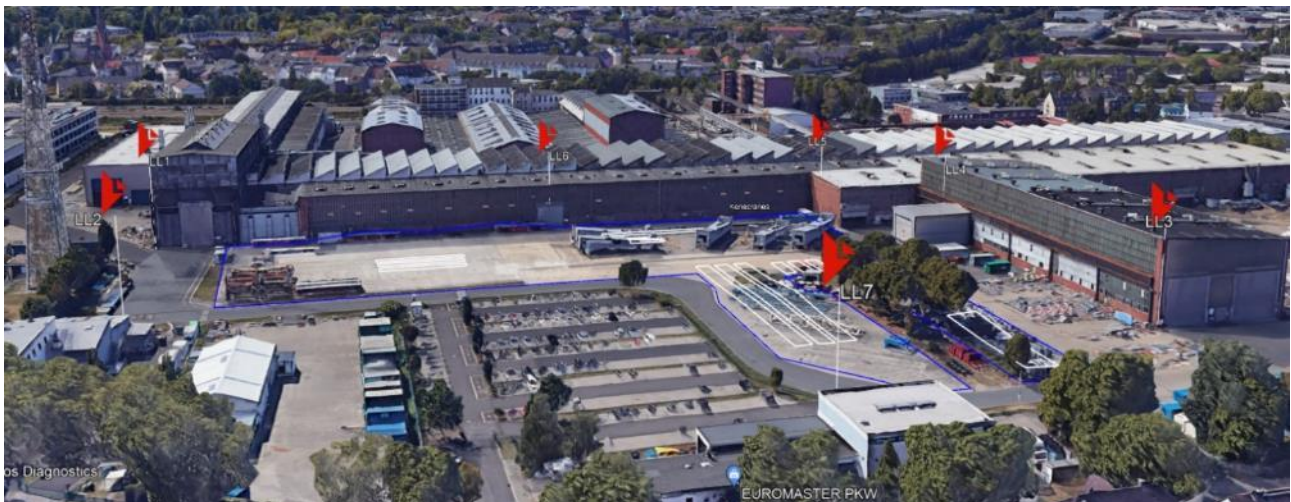
Figure 4-10: Outdoor Positioning Test – LocataNet 3D View
