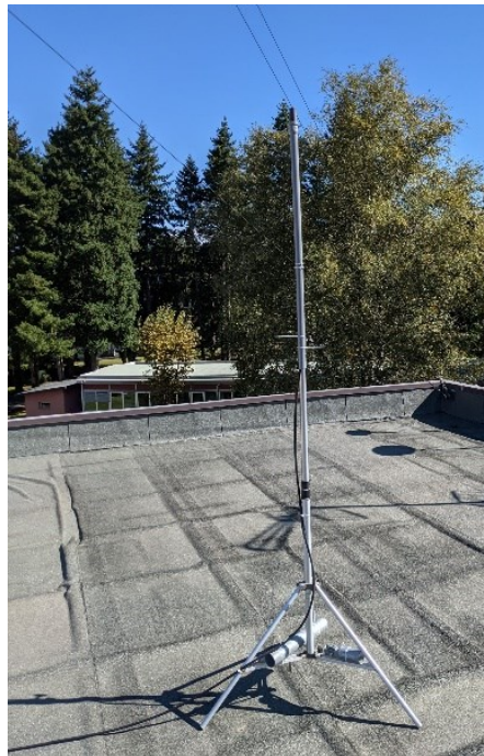
Figure 31 Satelles antenna on the roof of one of the JRC laboratory.
